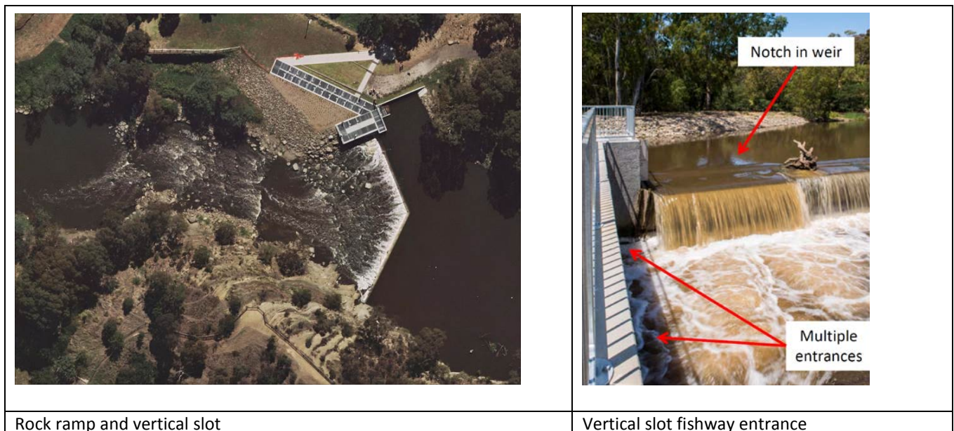
Figure 1: Dights Falls fishway complex: The rock ramp and vertical slot fishway (river flow direction is from right to left); and the two entrances to the vertical slot fishway and the weir notch to attract fish to the entrances
